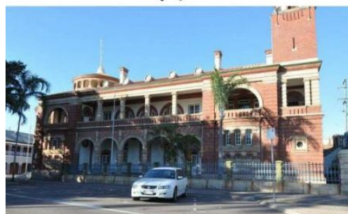
Figure SC6.3.5.33 Illustrates an undesirable outcome: former Customs House (The Strand, Townsville). Change of use to a private residence diminishes the associations and meanings of the heritage place
